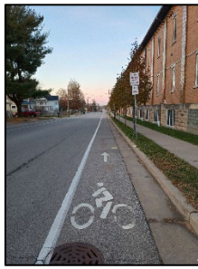
Painted bicycle lane along N East Ave (47%)
