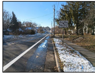
Painted bicycle lane along E Decker St (39%)
