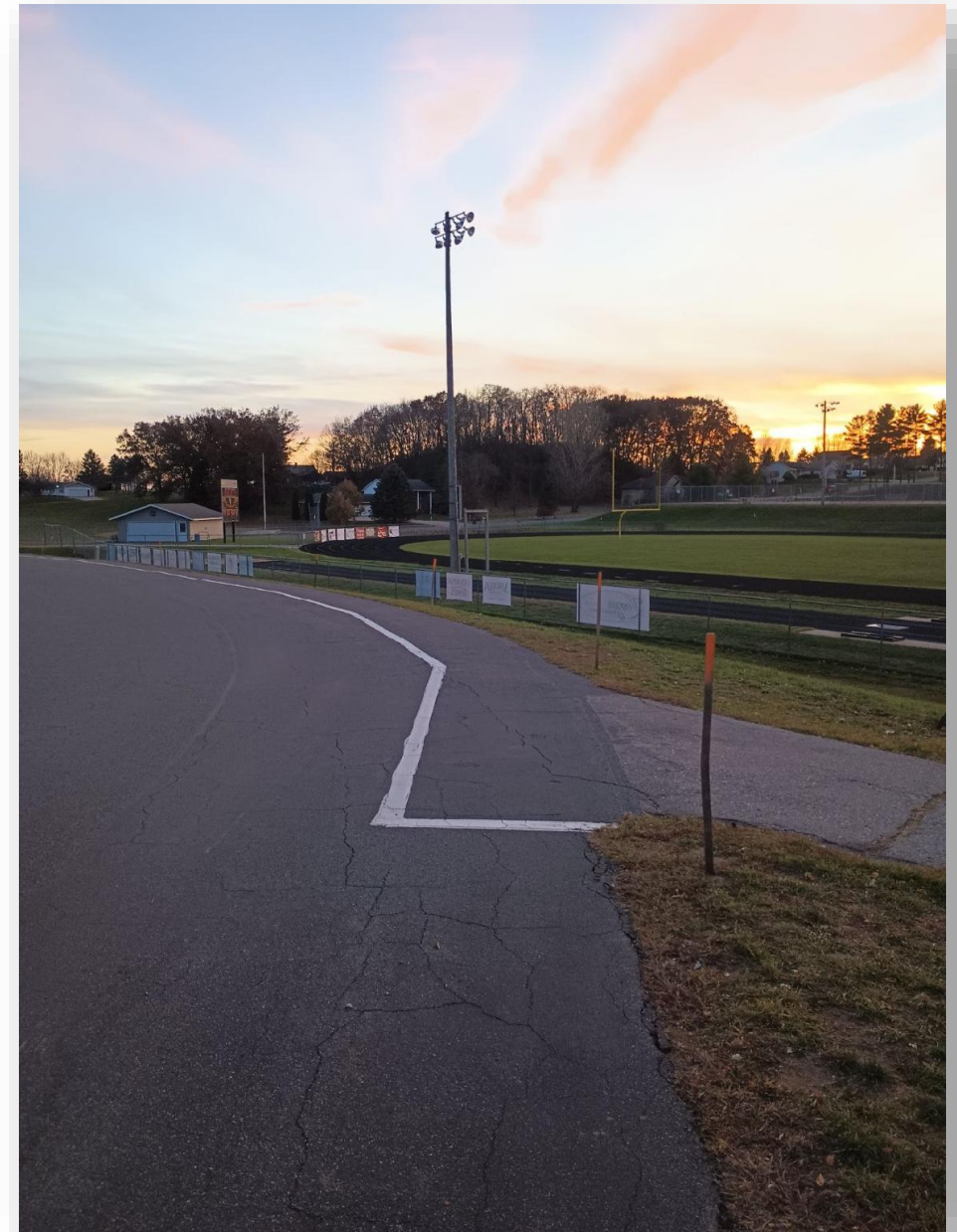
Painted pedestrian lane on Parkwood Trail
