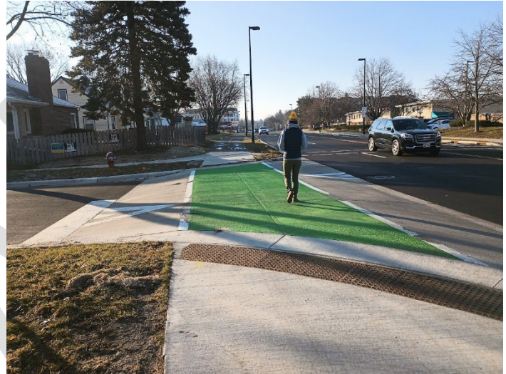
Figure 3.16. This speed table also functions as a raised crossing for a trail along an arterial street.
