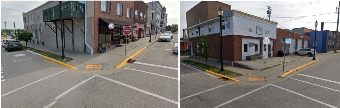
Figure 3.21: At the intersection of Rock Avenue and Jefferson Street (left) a catch basin has been placed upstream of the curb ramp, which better facilitates winter maintenance. At the intersection of Rock Avenue and Terhune Street (right), a catch basin has been placed downstream of the curb ramp, making this location more challenging for winter maintenance. Image Credit: Google
