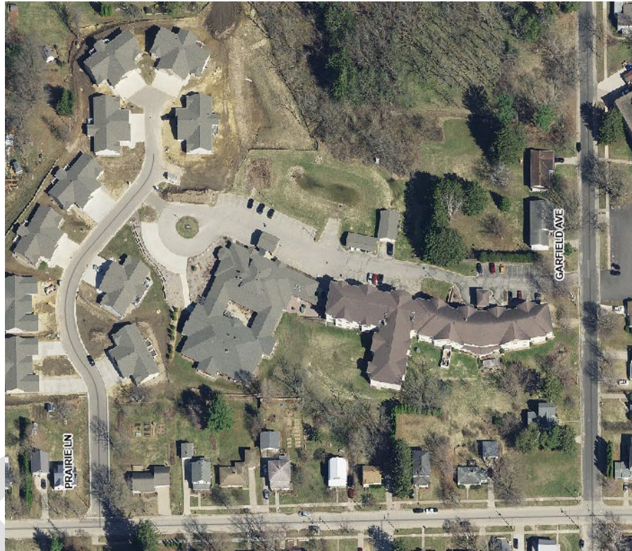
Figure 3.11: A recent retirement community development along Prairie Lane does not include sidewalks. Image Credit: Vernon County GIS
