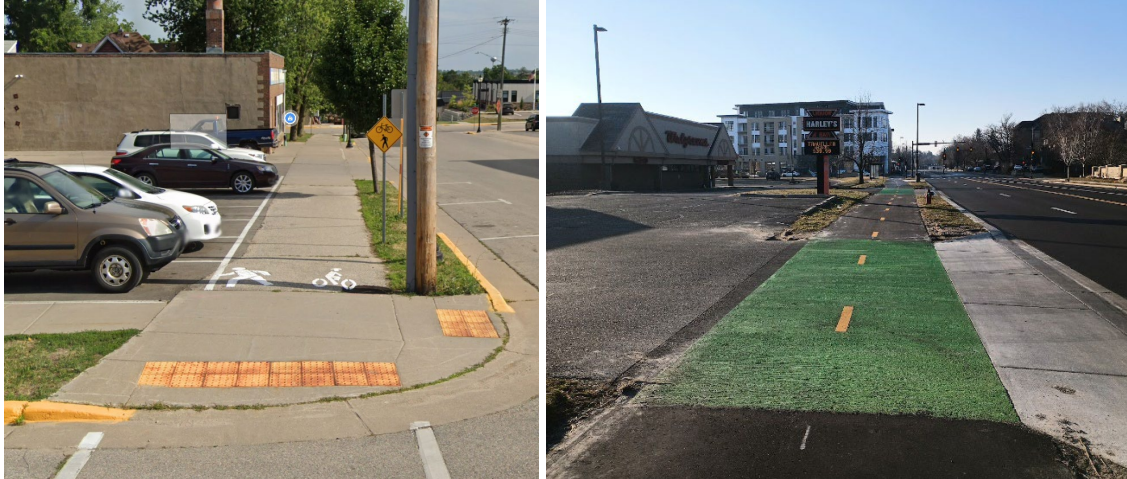
Figure 3.18: The Rock Avenue trail on the left does not include physical barriers to prevent cars from parking on the trail. The trail on the right includes both physical barriers and color differentiation to increase the visibility of pedestrians and bicyclists. Left Image Credit: Google
