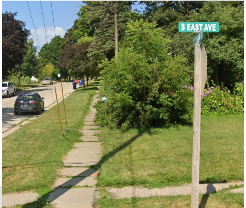
Figure 3.24: Vegetation can encroach onto sidewalks from the private property edge, making sidewalks impassable for many pedestrians including people with disabilities. Credit: Google
