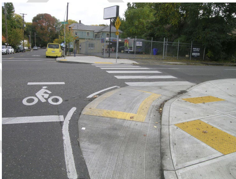
Figure 3.15: A truck apron can be used at a bump out to slow turning passenger vehicles but allow large vehicles to make turns without driving onto pedestrian waiting areas.
