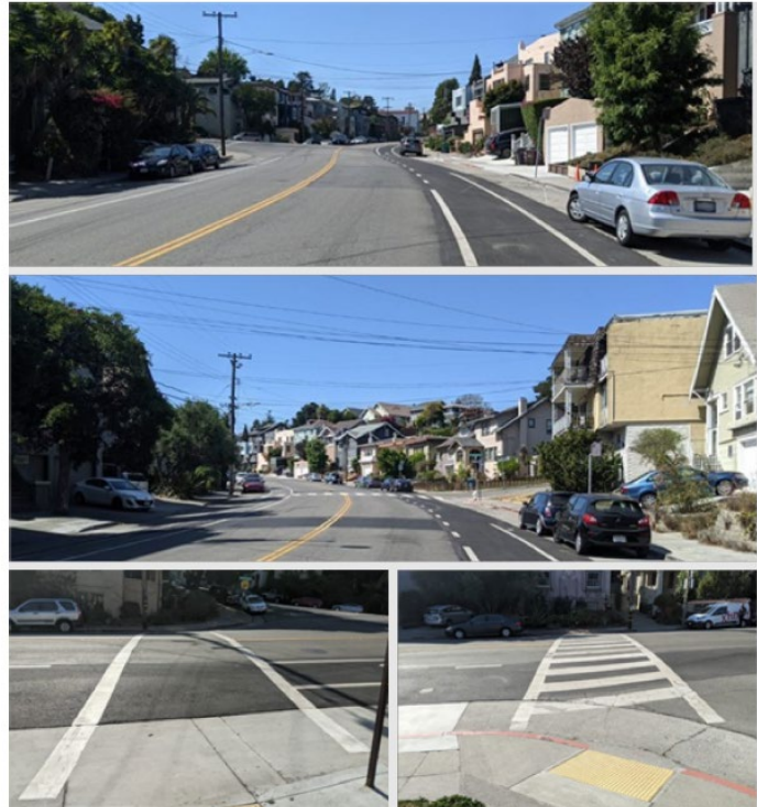
Figure 3.17: High visibility crosswalk (HVC) markings are more visible to motorists as the approach a crosswalk (see middle and lower right images). Credit: FHWA Crosswalk Marking Selection Guide
