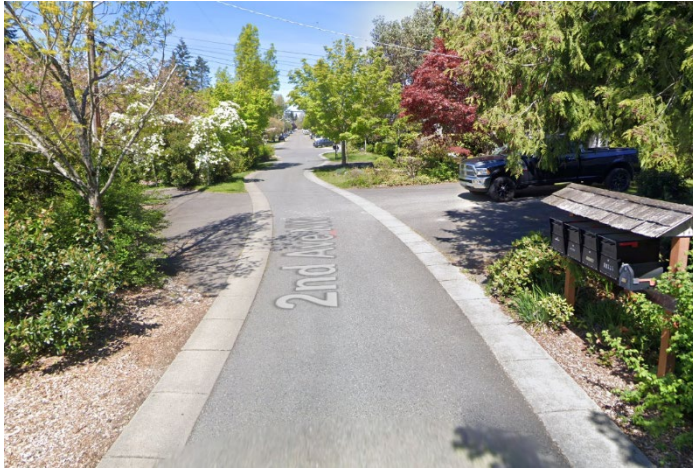
Figure 3.9: This 14' wide street in Seattle consists of 10' asphalt in the middle and 2' concrete strips on either side. Credit: Google
