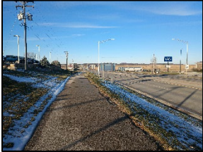
Shared use path along US Hwy 14/61 (76%)
