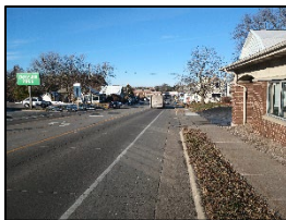
Shoulder along Main St (16%)
