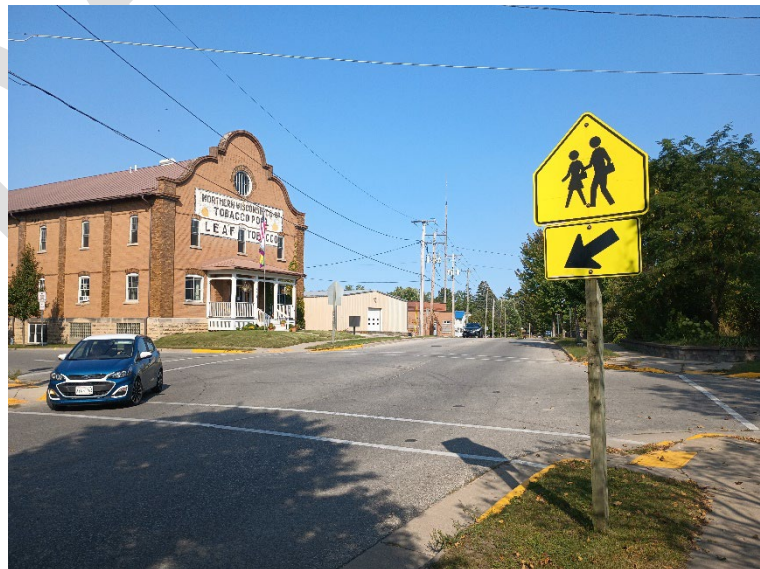
Figure 5.7: The intersection of Decker Street at lower left and middle (WI-56) with N East Avenue at left and right.
