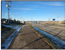
Shared use path along US Hwy 14/61 (80%)
