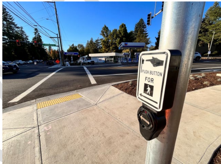
Figure 3.14: Push buttons should be placed parallel with associated crosswalks and include tactile arrows for people with disabilities. Credit: https://www.youtube.com/watch?v=UHS2VDrTuig
