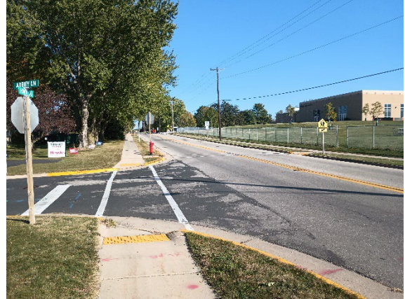
Figure 5.3: The intersection of Broadway Street at right (WI-56) with Abbey Lane at left.
