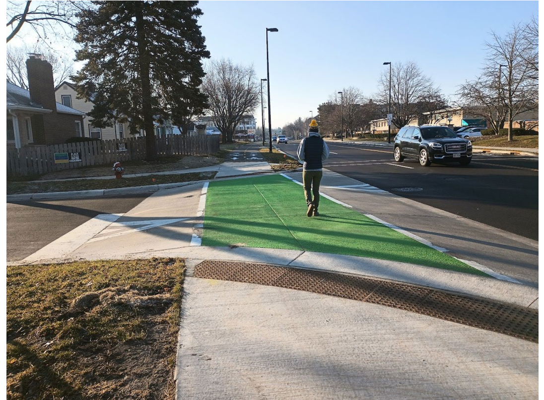
Green pavement and a speed table at a low volume street along Monona Drive in Madison.
