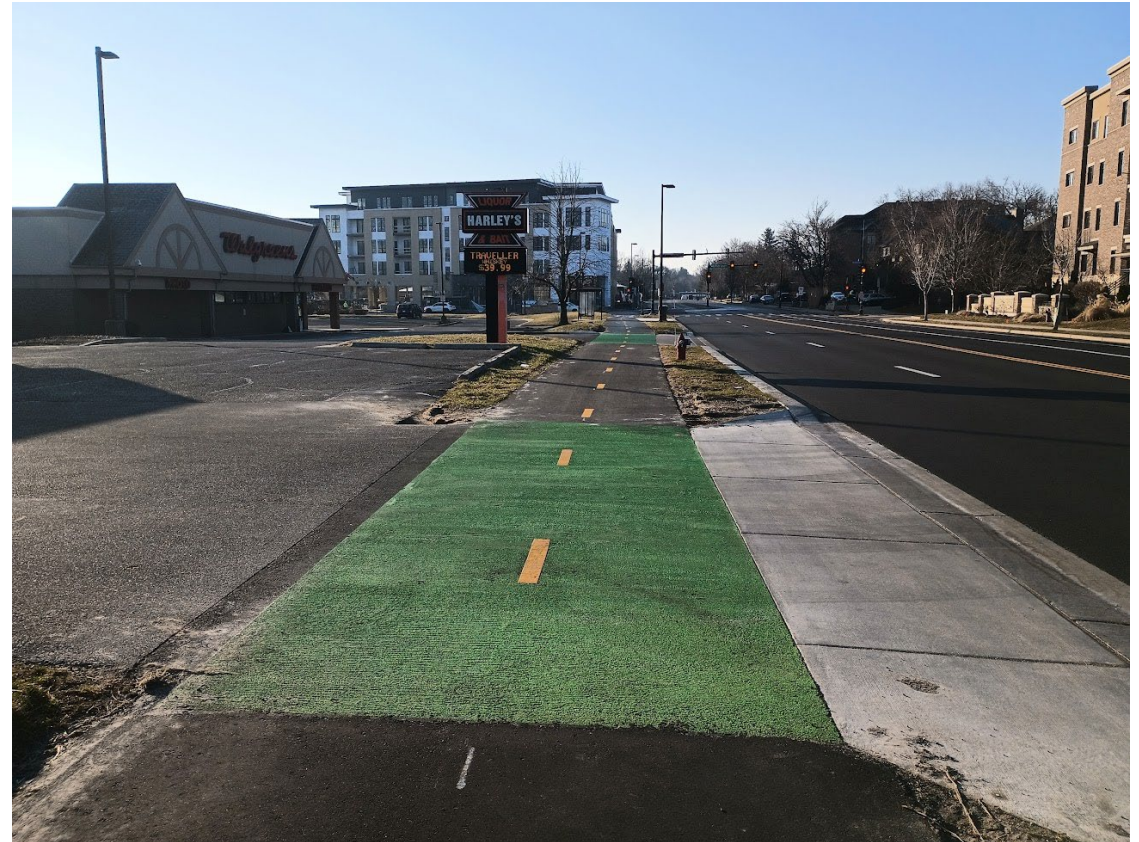
Green pavement at a driveway along Monona Drive in Madison.
