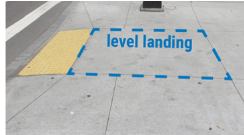
Example of a level landing
