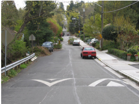
Figure 16. Speed humps, shown here on a residential street, are a traffic calming strategy.
