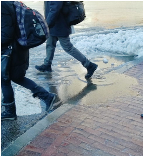
Poor drainage can lead to water pooling at curb ramps
