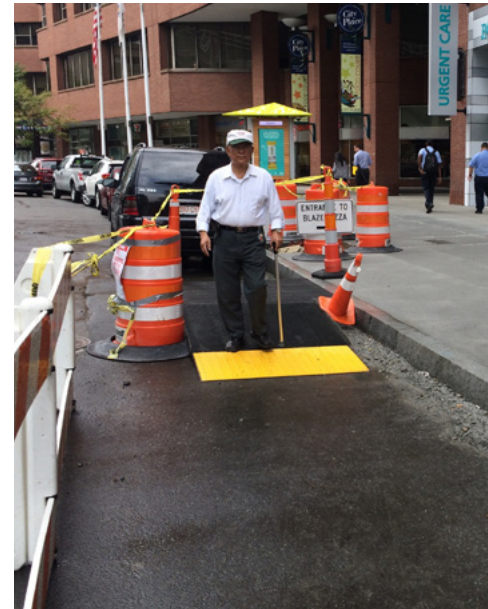
Pedestrians travel through a designated detour while construction activities are ongoing. A temporary accessible curb ramp is shown at right.
