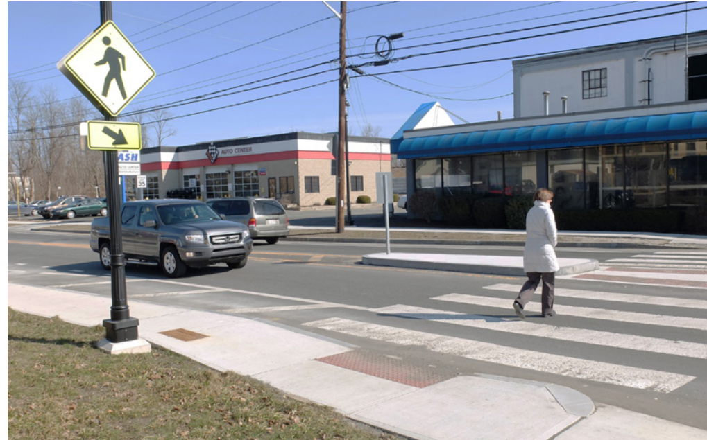
Walkable communities feature safe pedestrian crossings with ADA accessible curb ramps and signage indicating the crossing, such as on Pleasant Street in Northampton pictured above.
