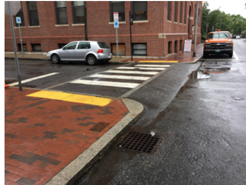
Figure 17. Raised crosswalks encourage yielding to pedestrians and reduce vehicle speeds.
