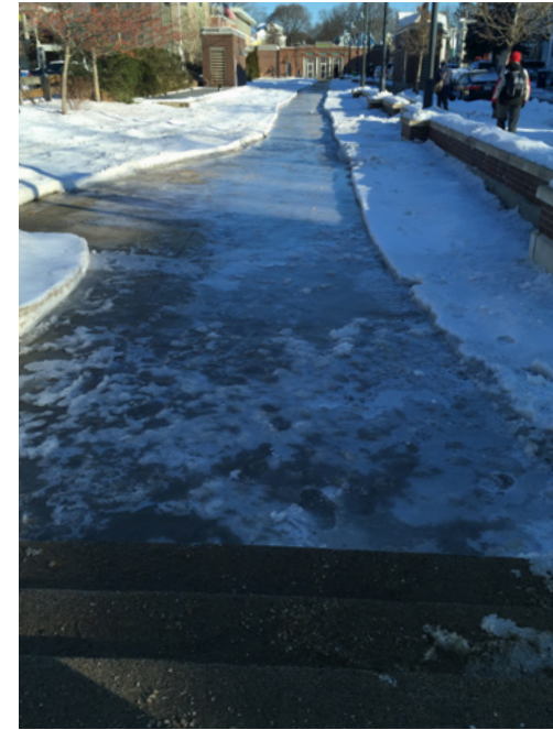
Walkways can become icy as a result of the freeze-thaw cycle.
